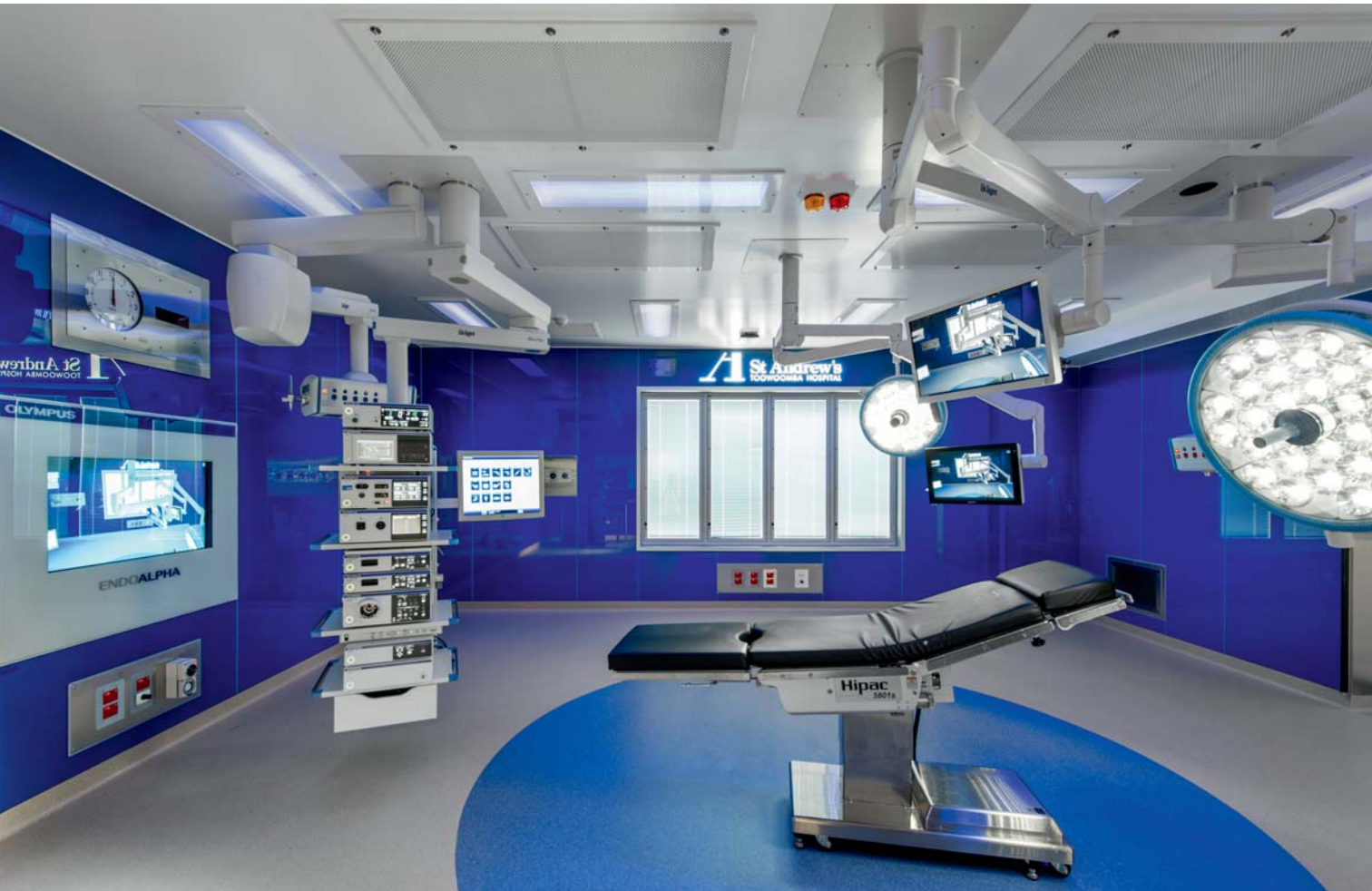
St. Andrew's Hospital, Toowoomba, Australia
